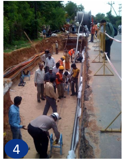
1. 33KV Feeder Bay at Raghunathgang - WBSETCL, 2. 132KV Transformer Bay at Bighati - WBSETCL, 3. 132 KV TRANSMISSION TOWER PROJECT AT MOGRA FOR WBSETCL, 4. Laying of 16 KM Double Circuit XLPE 220 KV Cable using various types of Rollers at Hyderabad - APTRANSCO
